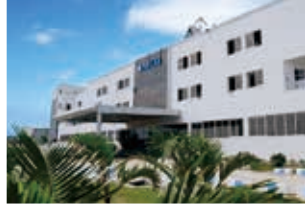
Rudrapur Plant (Green Building)
